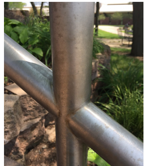
Welded stair railing near the Grote Building. Look for other welds on campus throughout your day!
